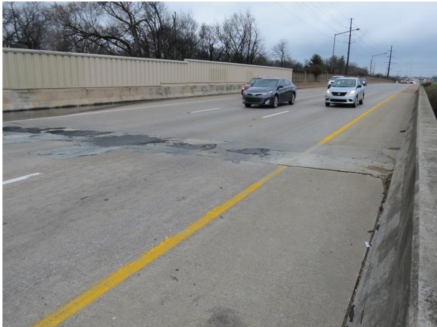
VIEW ACROSS TOP OF WEARING SURFACE WBL
